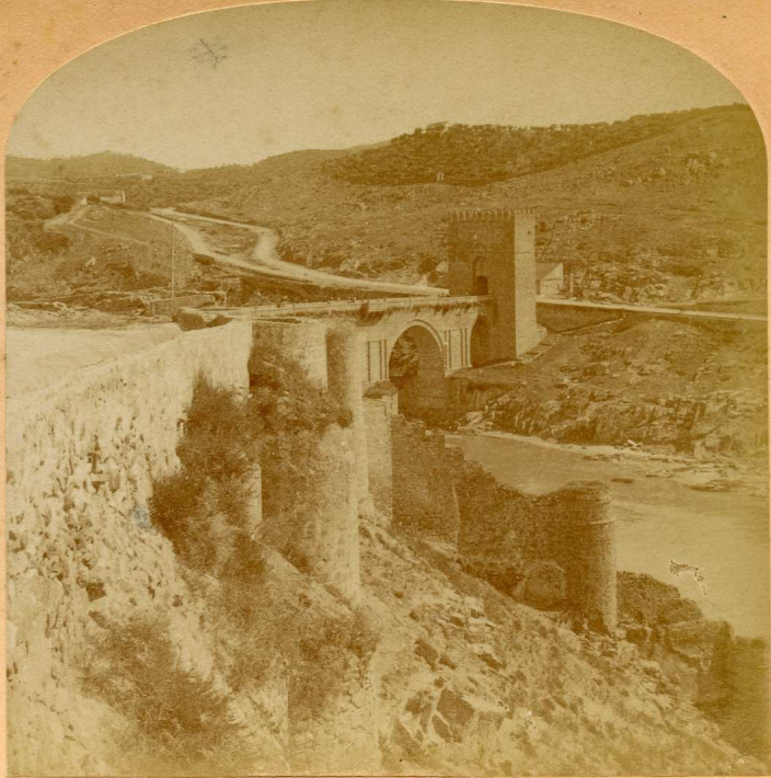
5829. San Martin Bridge, Toledo, Spain.
